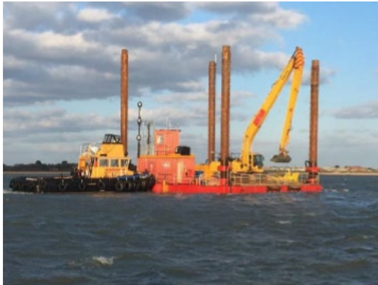
Plate 4-16: Example of a jack-up barge with backhoe excavator (Source: Equinor)
