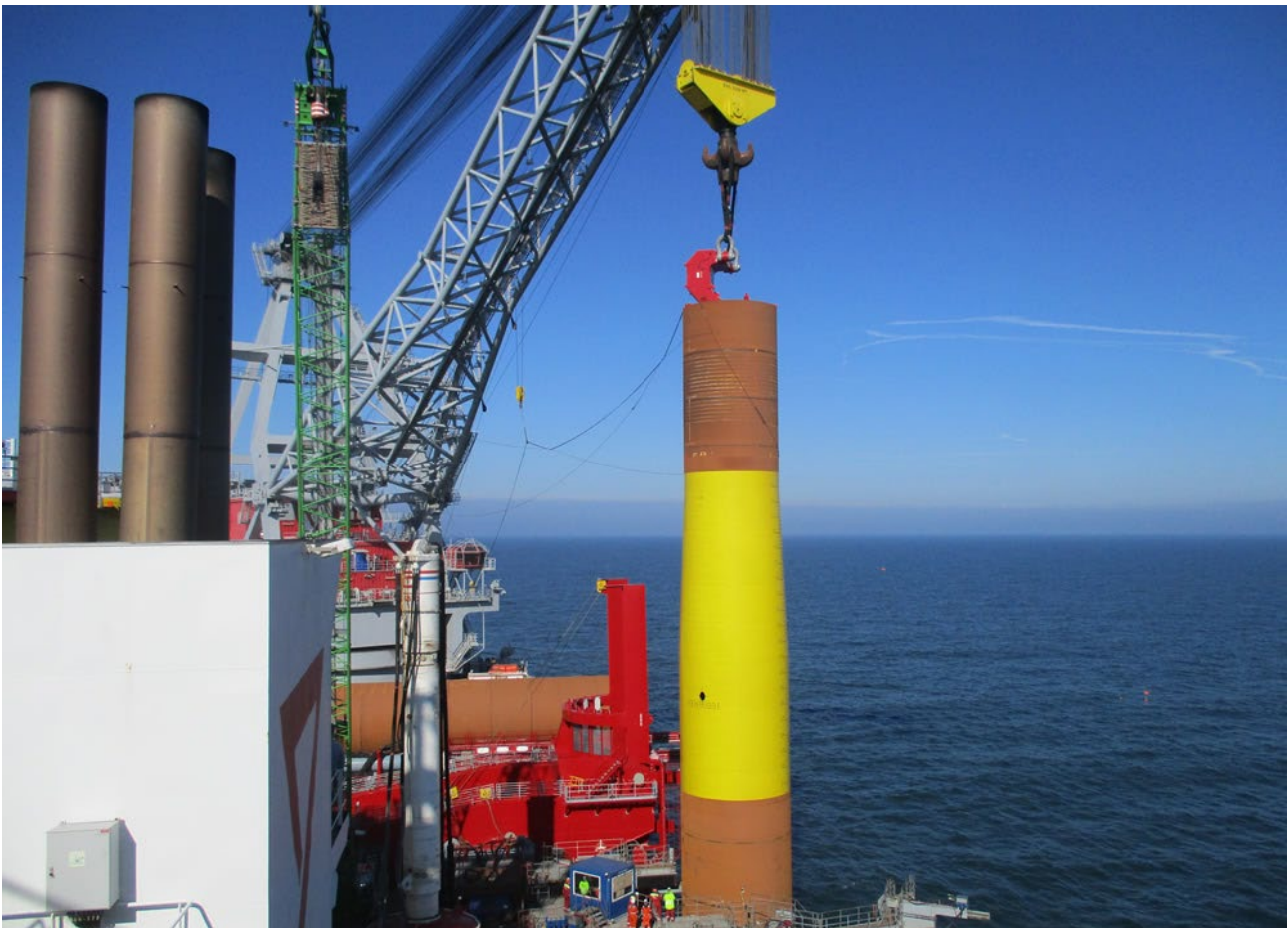
Plate 4-5: A monopile foundation being installed at DOW (Source: Equinor)
