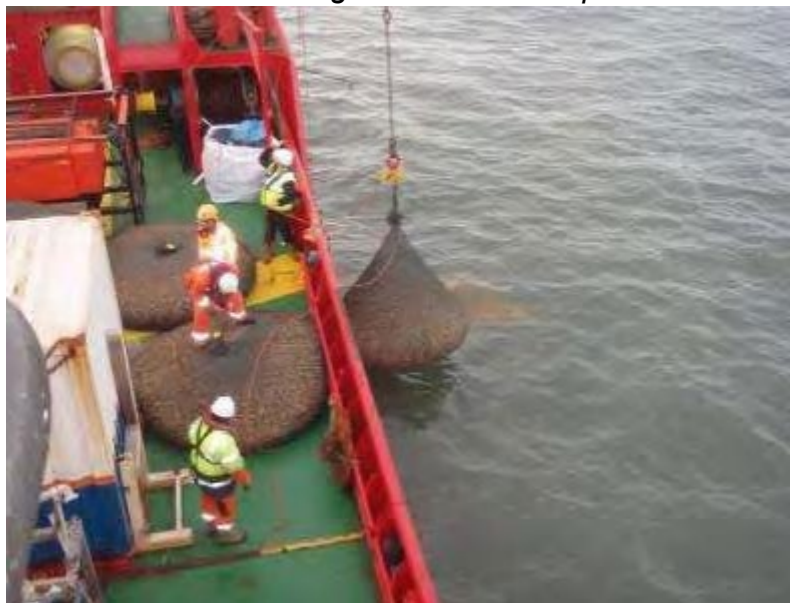
Plate 4-15: Rock bag installation (Source: Equinor)
